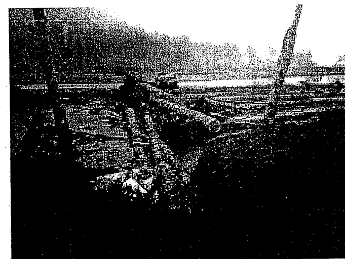
Figure 9.23: Engineered log jams. Engineered log jams (ELJs) can restore riverine habitat and in some situations provide effective bank protection.
