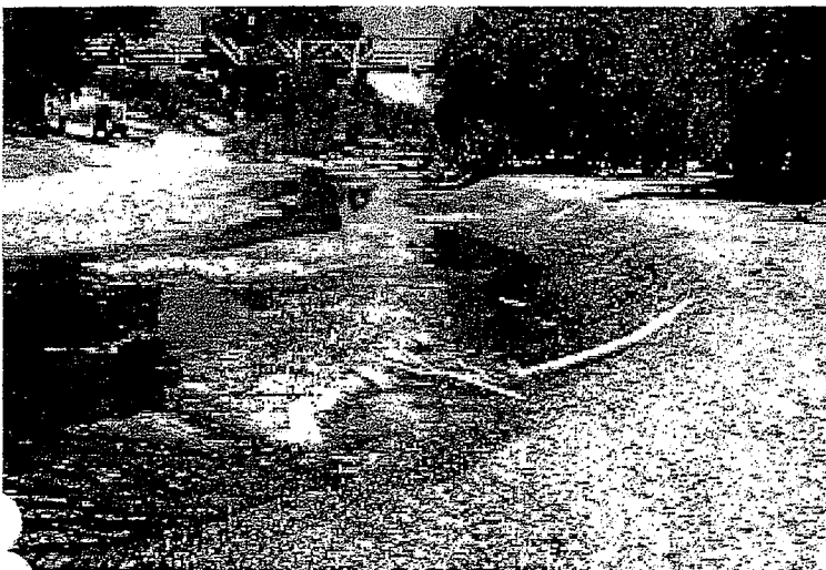
Figure 8.24: Low energy system with small bank angles. Bank angles need to be considered when using the tractive stress approach.
