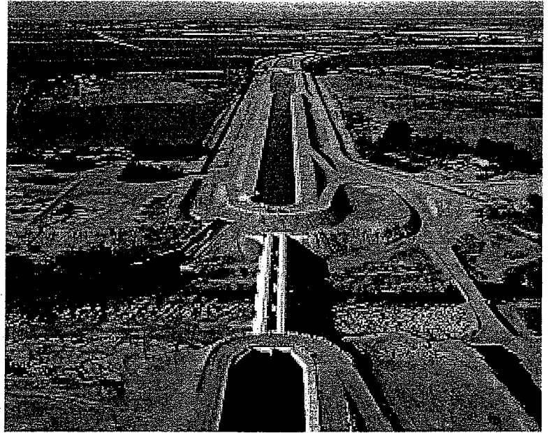
Figure 3.11: Stream diversion. Diversions are built to provide water for numerous purposes, including agriculture, industry, and drinking water supplies.
