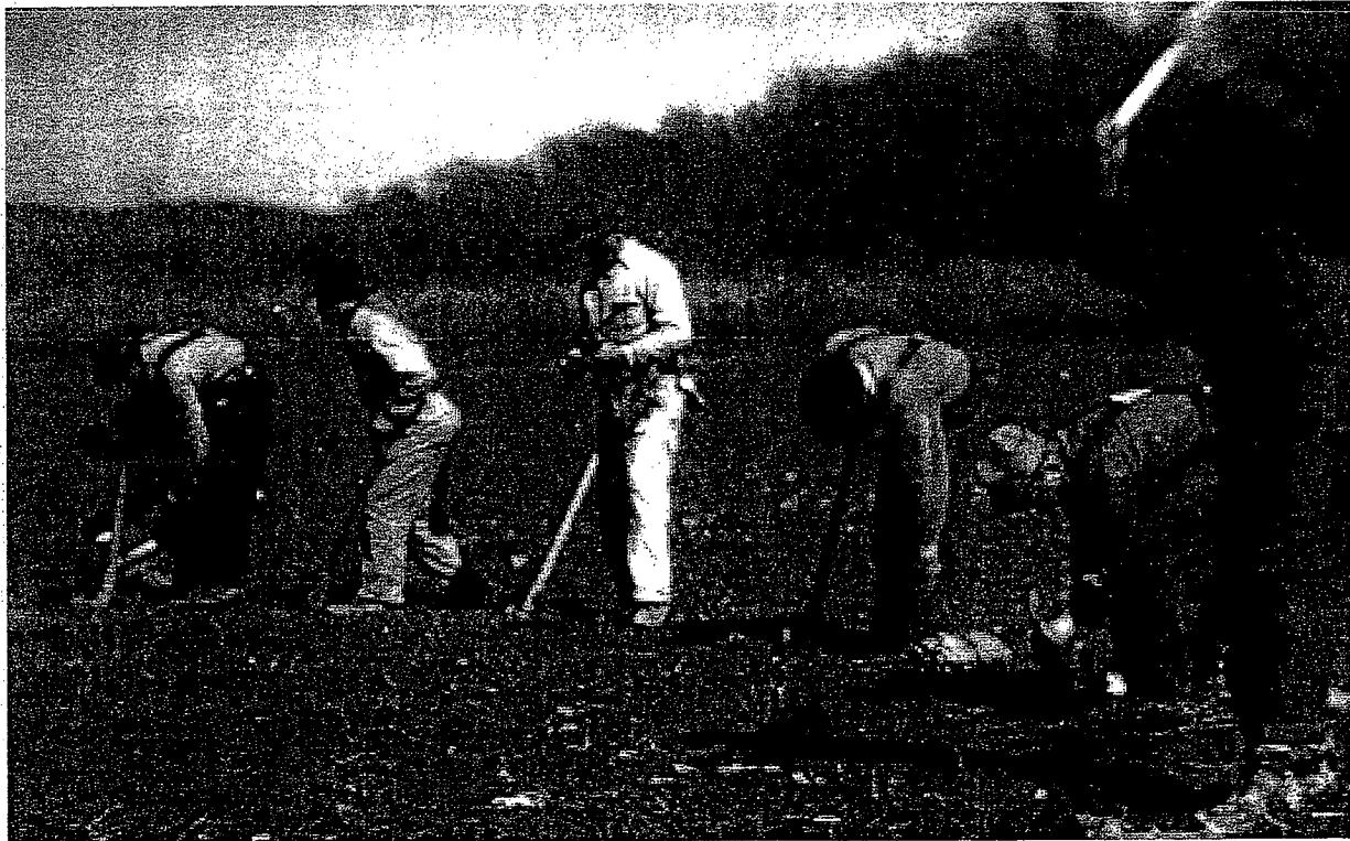
Figure 8.13: Kentucky Reservoir watershed, 1943. Planting abandoned farmland with trees.
